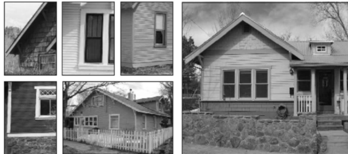
Local examples of the use of horizontal lap siding and wood shingles, note the appropriate use of color on the siding and trim. Also note window type, proportions, and details.
